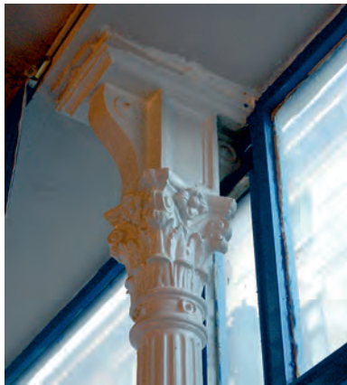
Fig. 24. Detail of cast iron column – extension. 8, Covaci Street.
