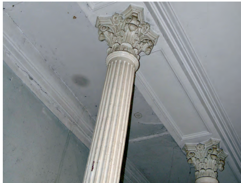
Fig. 11. Detail of isolated cast iron column. Armis Petrovici property, arch. P. A. Gottreau. 27, Lipscani Street.
