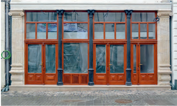
Fig. 7. Shop window with access opening framed by cast iron columns and protected by exterior roller shutter. Façade of. 42, Franceză Street.
