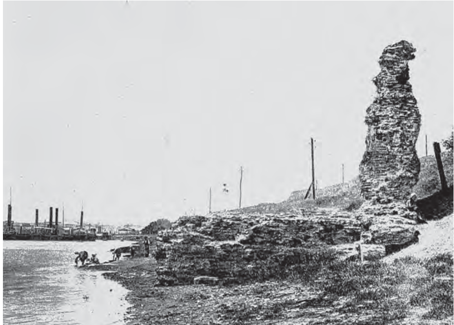
Fig. 1. Abutment pier on the Romanian Bank. Al. Antoniu, 1904.
