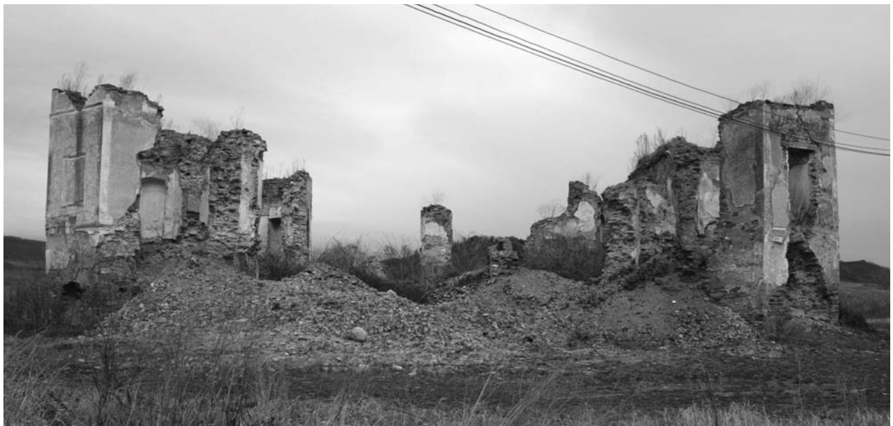
Fig. 8 The collapse of the southern façade. Photo: November 29th, 2010.
