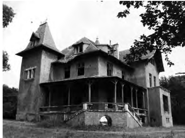
Fig. 10. The Large Castle. North-west view. June 2009
