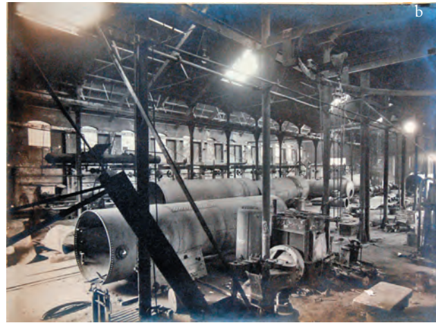
Fig. 18. Interior views from the workshops building. The roofing is made of metallic trusses that discharge on the cast iron pillar (Societatea f. a., BCUB, Unitatea Centrală, VI77/16).
