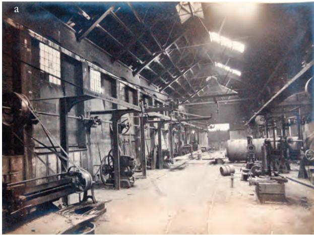
Fig. 18. Interior views from the workshops building. The roofing is made of metallic trusses that discharge on the cast iron pillar (Societatea f. a., BCUB, Unitatea Centrală, VI77/16).
