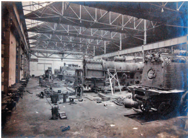
Fig. 19. Interior view from the workshops building (Societatea f. a., BCUB, Unitatea Centrală, VI77/16).
