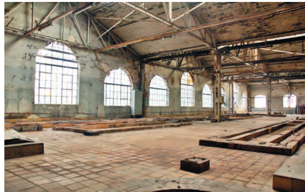
Fig. 22. Interior view of the building oriented towards the Carol Park, presently unused.
