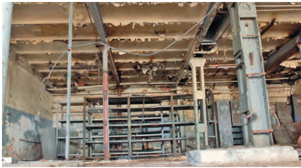
Fig. 25. Interior of the semi-basement. The space is covered with small brick vaults and laminated profiles supported by beams and composite pillars.
