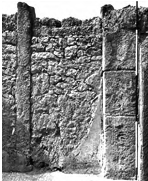
Fig. 7. Opus Africanum at the Punic block in the late period in Byrsa Hill. We can notice the large vertical blocks between which smaller horizontal rows of blocks were bound (Krings 1995, PL. 23).
